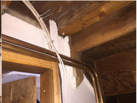
Photo 18: The wall on the hall side of the cupboard is a non structural stud partition, and the stair void trimmer beam spans across the hall to the kitchen wall
