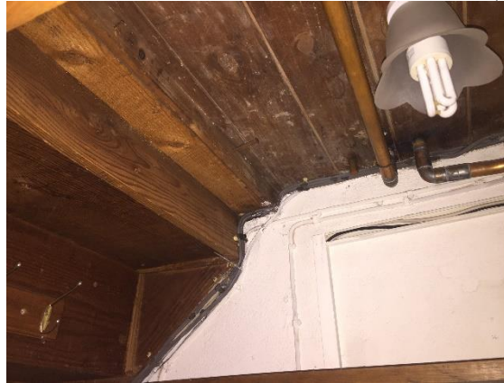
Photo 17: The 1 st floor stair void trimmer beam spanning onto the blockwork wall
