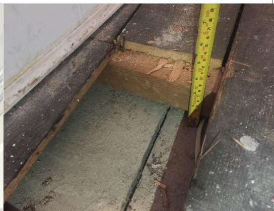
Photo 26: The raised floor is approximately 100mm above the original floor at the proposed lift position
