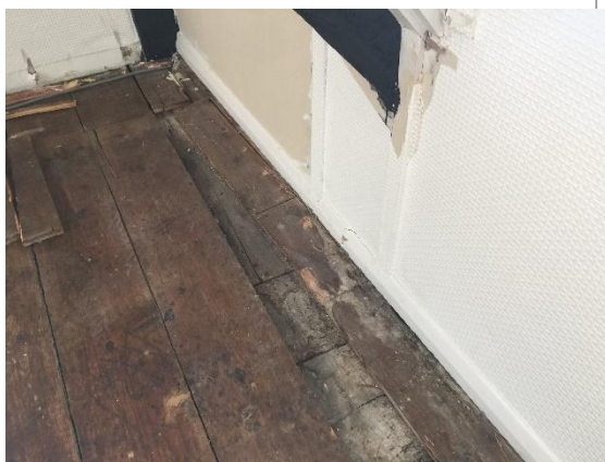
Photo 27: The joisting and boarding in the second floor has previously been modified and trimmed in modern joists between the two roof trusses
