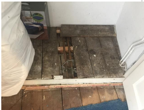
Photo 25: The first floor has a modern false floor installed above the original timber floor boards – presumably to level the floor
