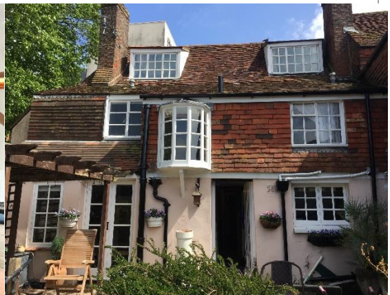
Photo 20: The rear elevation – right kitchen window to be converted into a door opening by removing the lower element of wall below the window
