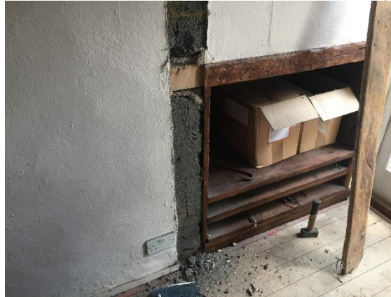
Photo 13: The modern blockwork wall below the ground floor stair landing
