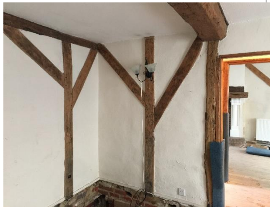
Photo 19: The location of the proposed new openings from the hall into the front left room and also in the wall from the front left room into the kitchen – the timber beam and post below are structural but the remainder of the timber around the walls in the photo are superficial and have been surface mounted onto the walls
