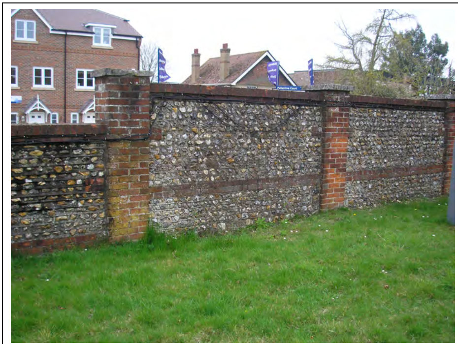
Photograph 10 - Brick and Flint Wall
