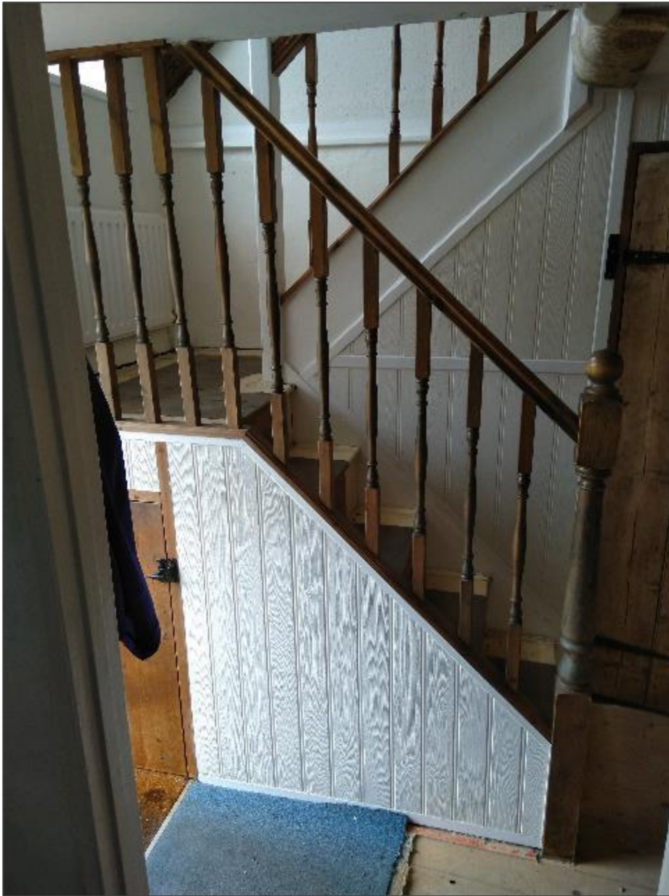
Plate VIII: Softwood timber staircase to half landing
