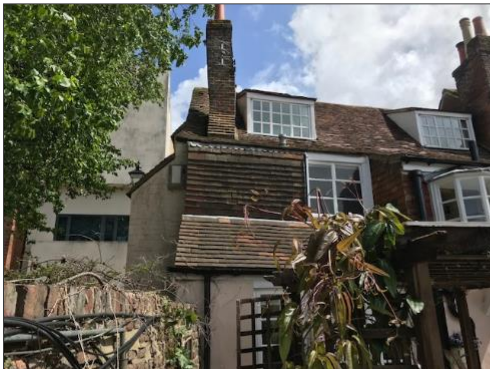
Plate II: North end, Rear (West) Elevation. Tile hanging to First Floor.
