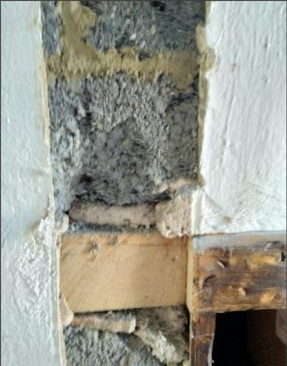
Plate X: Concrete blockwork to north wall of stairwell
