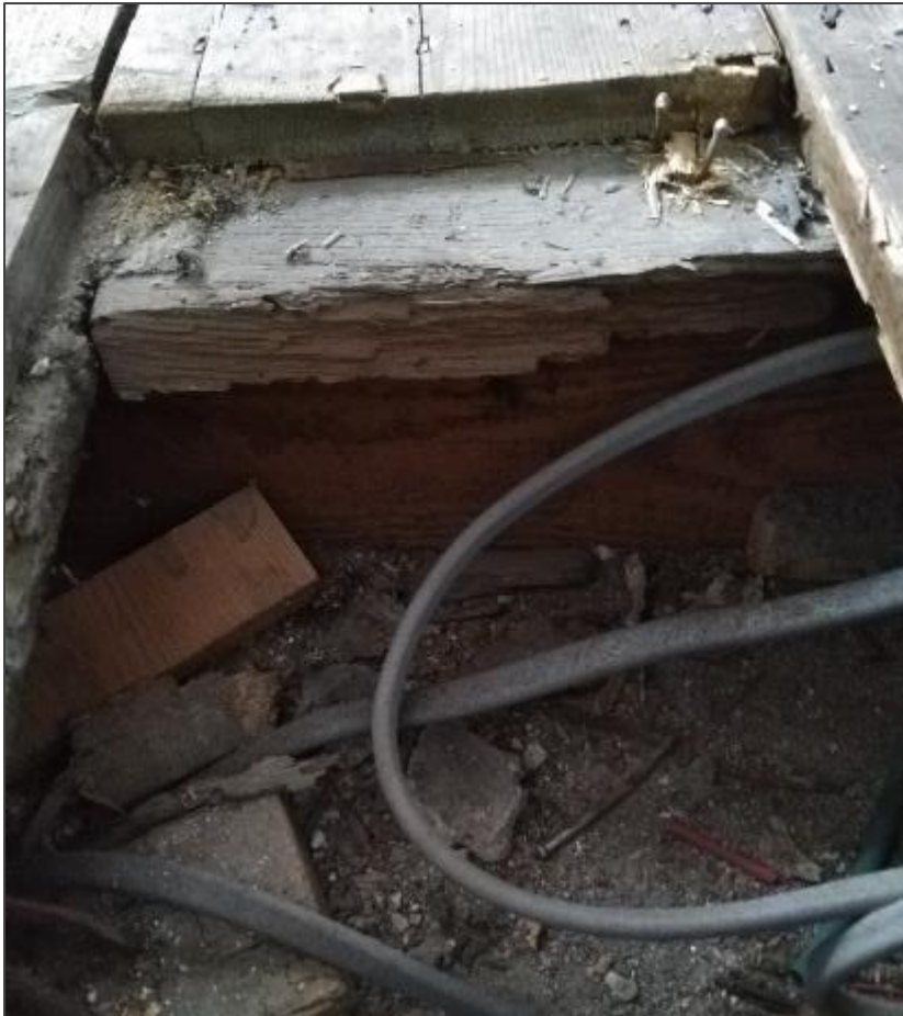
Plate XXII: Attic Floor, re-used boards overlaid with new. Modern joists adjacent staircase.
