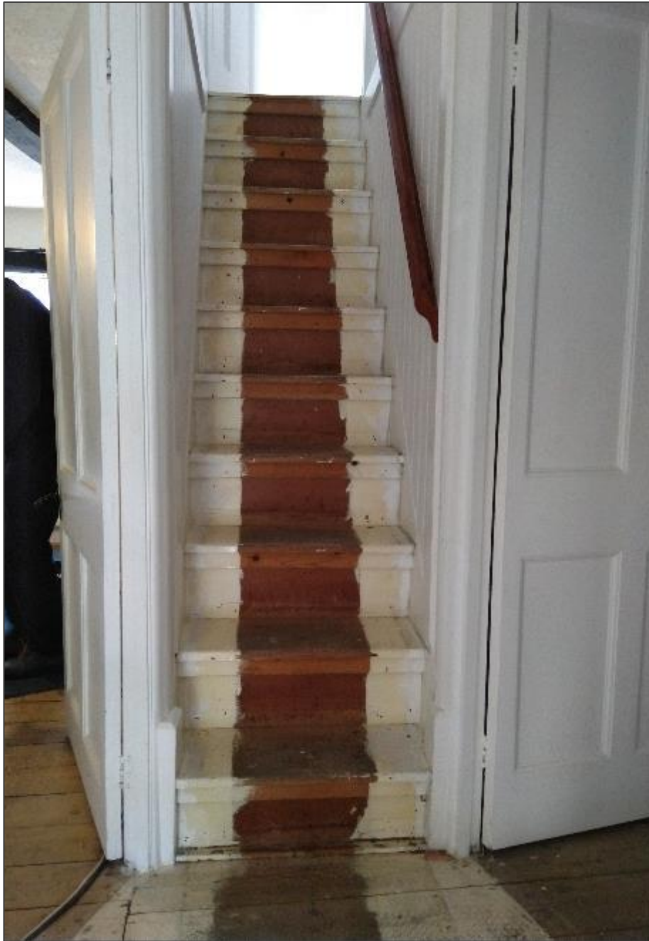
Plate XVIII: Staircase from First to Second Floor level (view from West).
